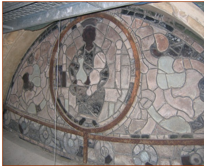
© CSM 2007 – detail of the rose window of the South Portal as seen from the outside during restoration work.
